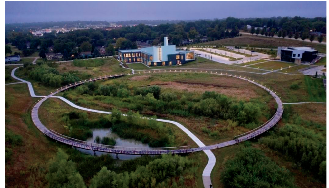
An overhead view of Abraham's Bridge on the Tri-Faith campus.
